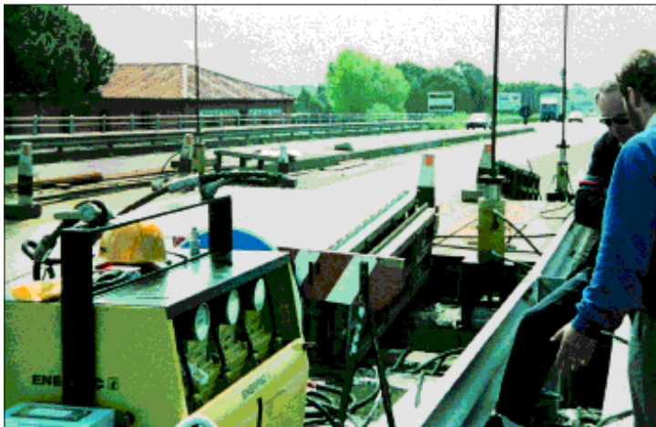
◀ Here a bridge deck is being re-leveled after major maintenance work.
